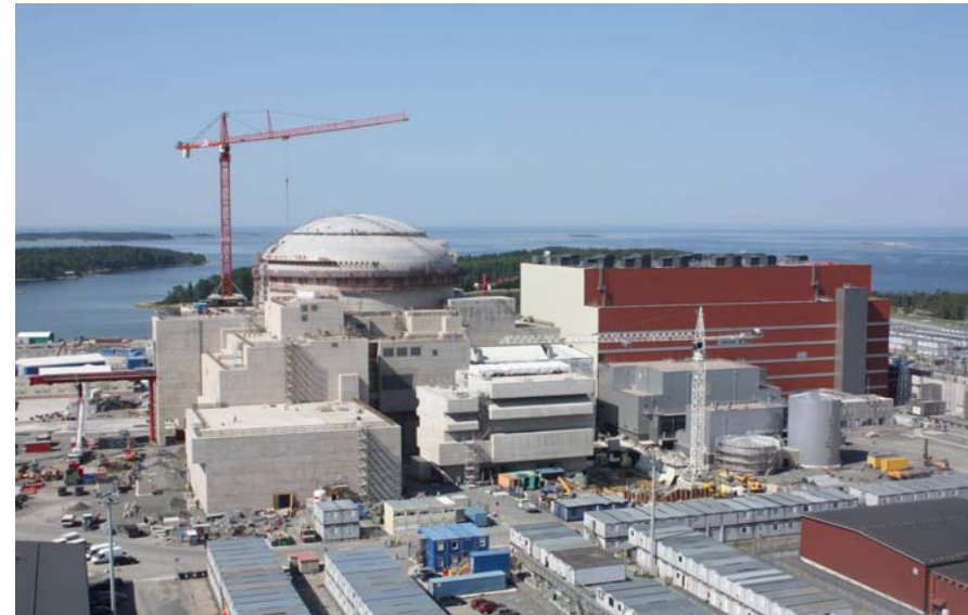
EPR™ reactor construction site, Olkiluoto (Finland). 2011, July
