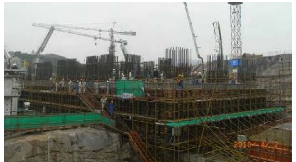
TSNP phase I NI raft concrete pouring
