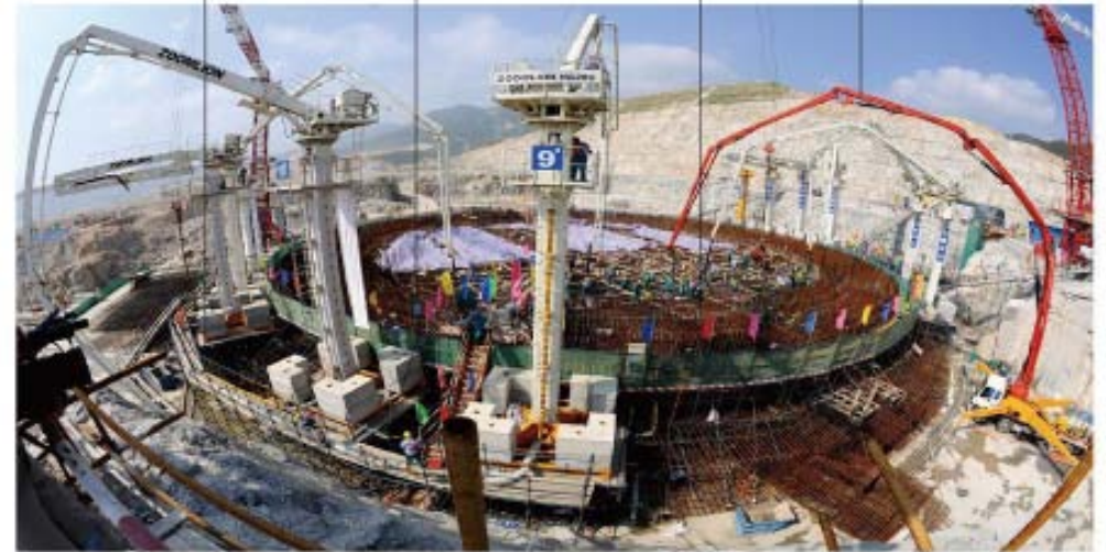
TSNP phase I NI raft concrete pouring
