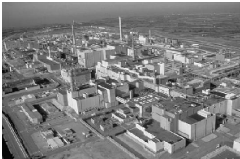
Figure 7.1. Aerial view of the La Hague UP3-A Plant (Source: COGEMA – France)
