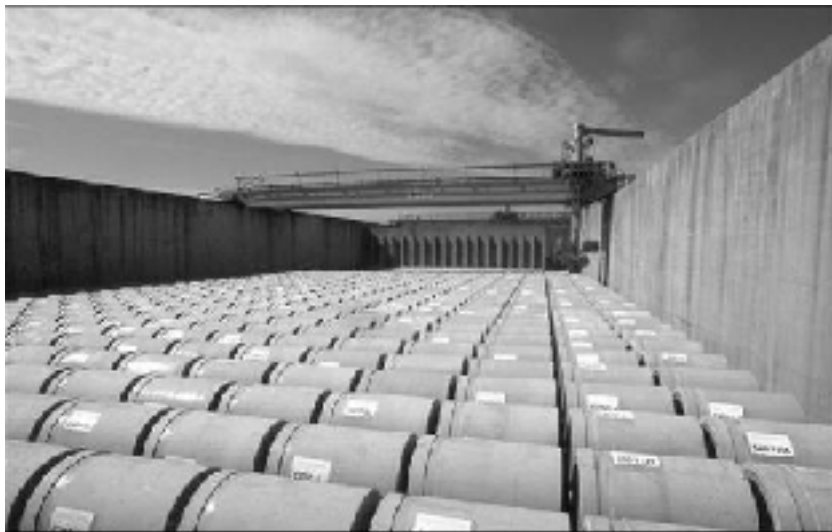
Figure 2.18. EDS LLW drums storage at La Hague (Source: COGEMA – France)
