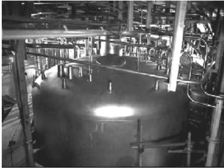
Figure 2.15. Fission products solution tank in the R7 facility (Source: COGEMA – France)
