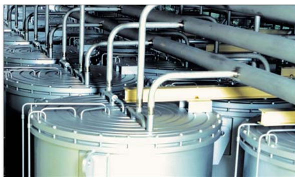
Cascade of centrifuges at Rokkasho-mura in Japan.
