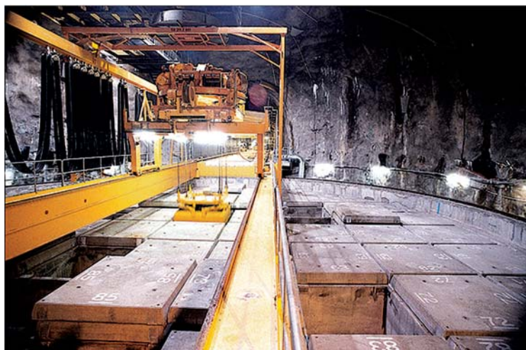
Repository for LLW and ILW in Sweden.
