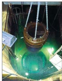
Removal of the Belgian BR3 reactor pressure vessel for further dismantling.
