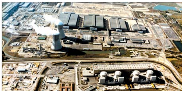
Uranium enrichment plant at Tricastin, France. This enrichment plant alone is large enough to more than meet the needs of all nuclear reactors in France.
