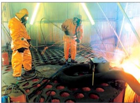
Top biological shield being dismantled using a thermic lance process at the Windscale Advanced Gas-cooled Reactor Dismantling Project.
