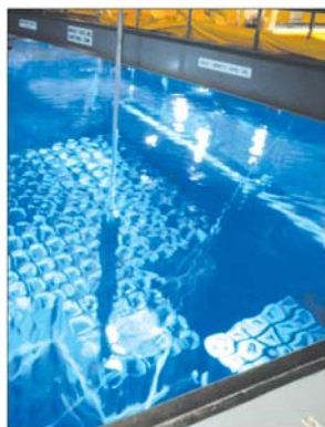
Typical spent nuclear fuel storage pool.
