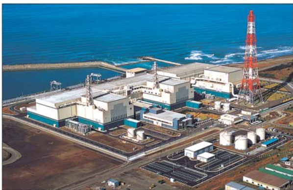
Construction of units 6 and 7 at the Kashiwazaki-Kariwa nuclear power station in Japan was accomplished in under six years.
