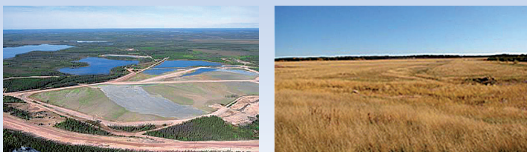
Cluff Lake tailings management area (TMA) prior to decommissioning (left) and after decommissioning and re-vegetation (right). During the operational life of the Cluff Lake mill, all tailings and contaminated water generated at the site were transferred to the TMA for disposal and treatment. Decommissioning in 2001 and 2003 included placement of a 1 m till levelling course over the tailings storage areas to minimise radiological hazards and dust emissions, as well as to promote tailings consolidation.
