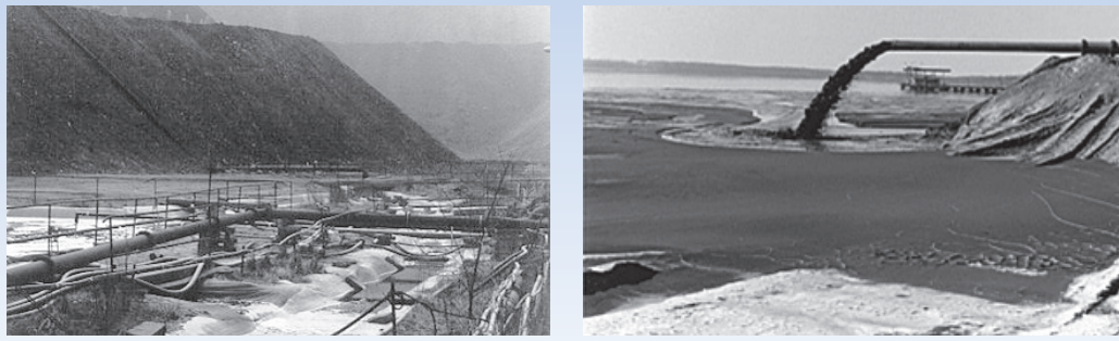
Helmsdorf tailings disposal area during operations: tailings were deposited in a shallow valley adjacent to the processing plant, contained by two dams constructed of waste rock. No bottom liner for groundwater protection was installed prior to operation and little consideration was given to the potential impacts from leakage or a dam failure on communities located downstream of the impoundment.
