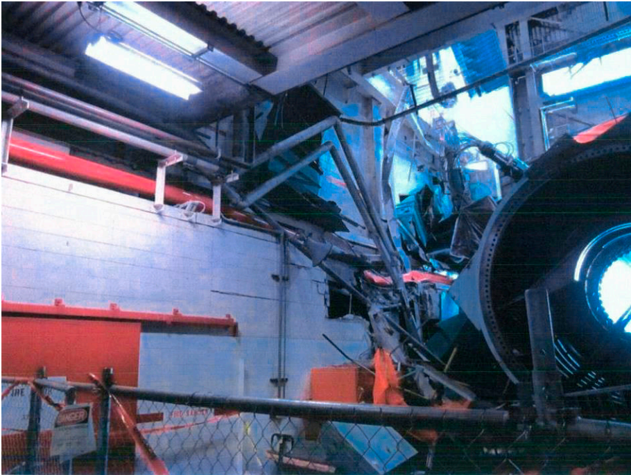
FIG. 2. Dropped stator (partially shown on the right).
