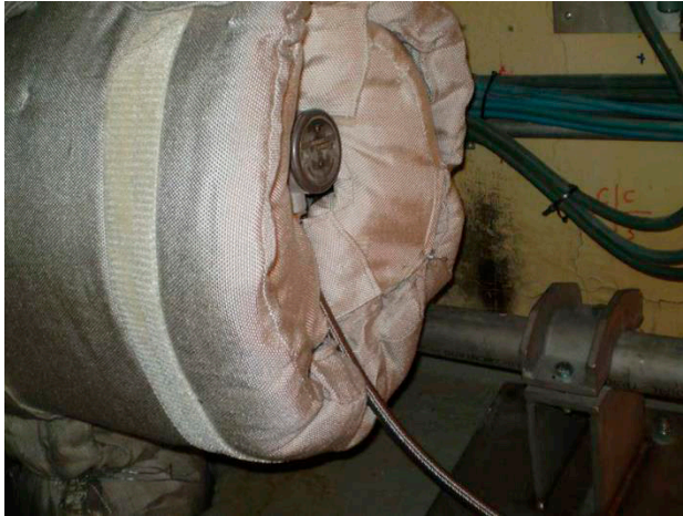
FIG. 4. Proper insulation installation.
