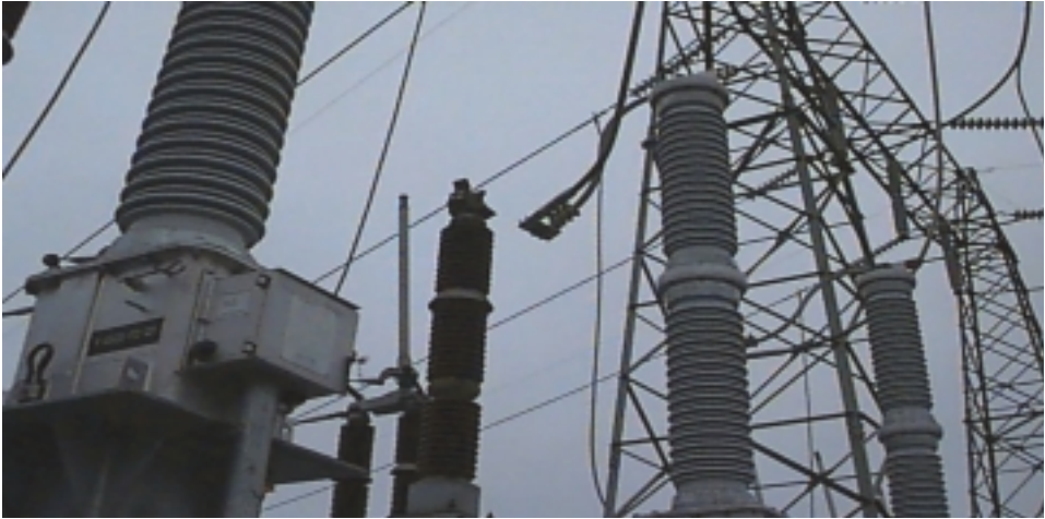
A 230 kV conductor on the jaw side of a disconnect switch was found broken and hanging freely (source: COG, Canada)
