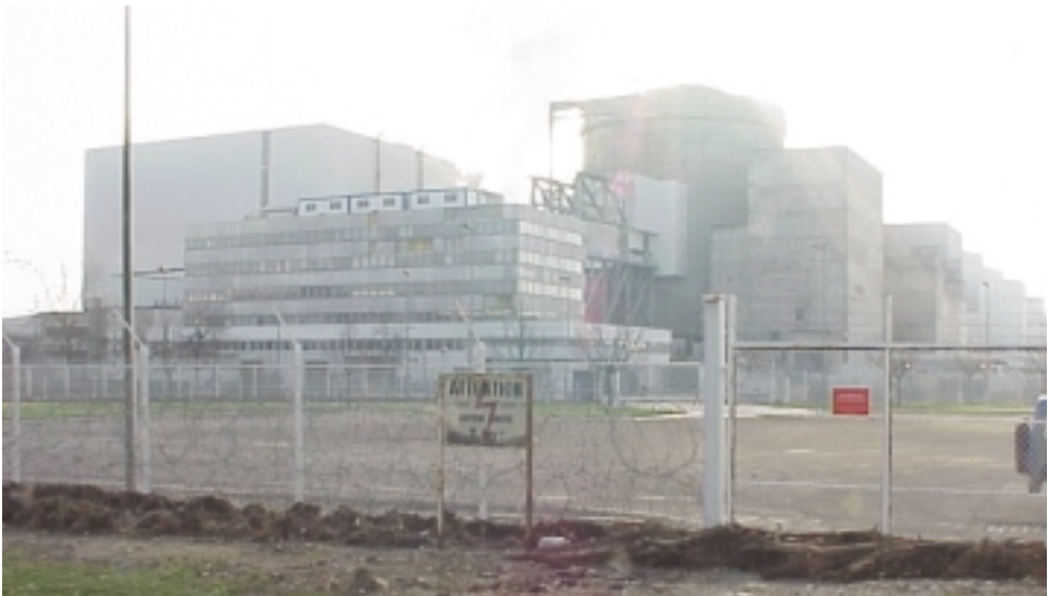
Debris accumulation outside the chain-link fence indicates water level above the site platform (source: IRSN, France).
