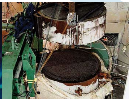
Dismantling of a steam generator using an "ice sawing" technique.
