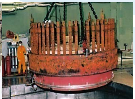
Dismantling of the RPV – transporting the flange.
