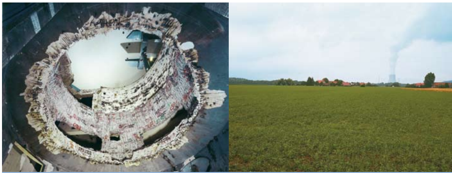
Dismantling of the biological shield.
