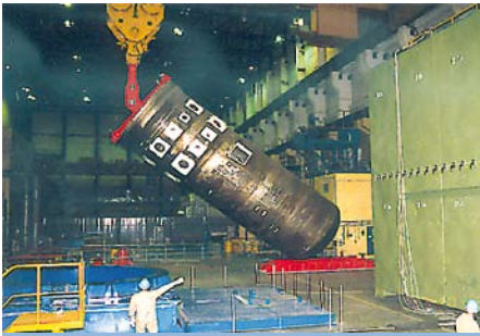
Removal of a reactor pressure vessel.
