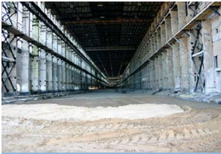
Empty turbine hall.
