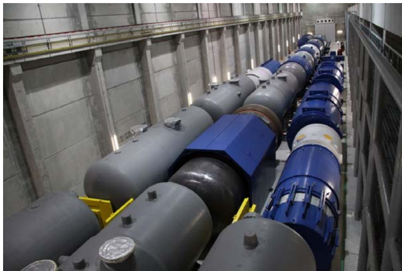
Figure 4: North Interim Storage Facility
