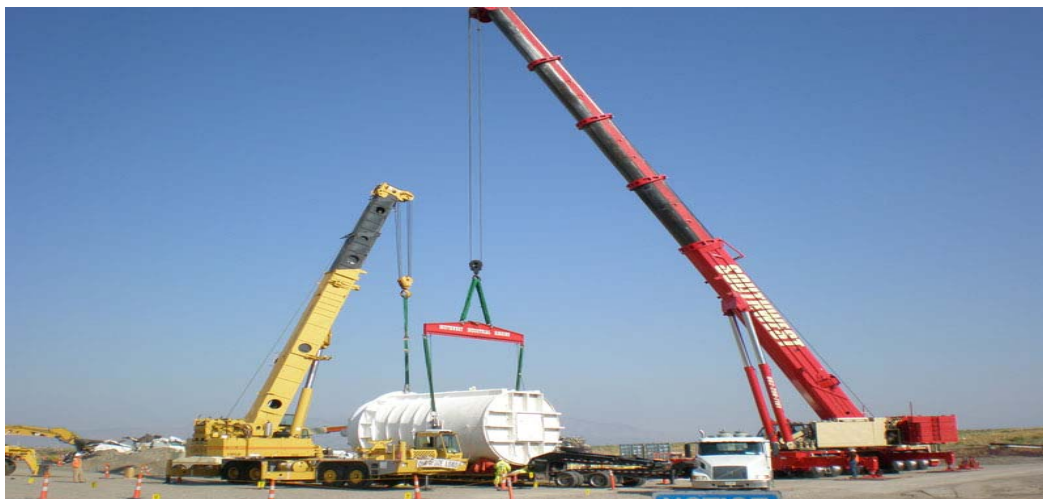
Figure 5: Removal of the PBF vessel.
