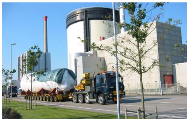
Figure 2: Steam Generator at Ringhals NPP
