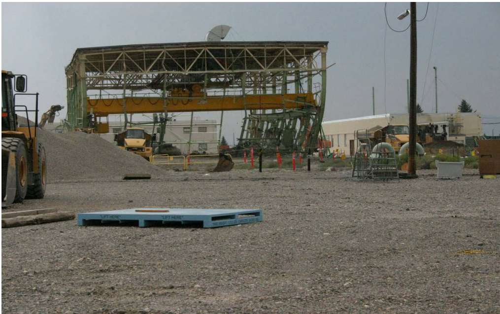
Figure 3: Building TRA-642 pullover
