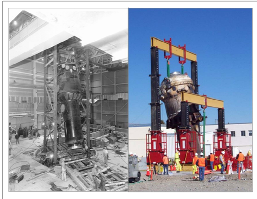
Figure 4: Installation and removal of the ETR vessel
