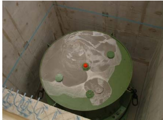
Figure 4: PRV head at its disposal location, after grouting
