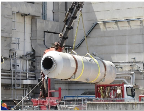
Dismantling of components.
