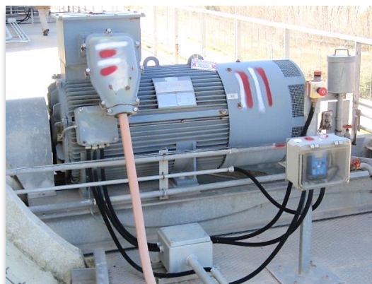
Discharge of components prior to dismantling.
