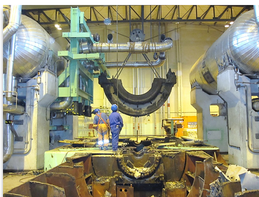
Dismantling of the turbine components.
