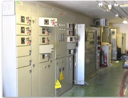
New electrical building.
