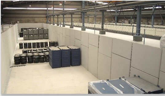
Waste storage upgrading.
