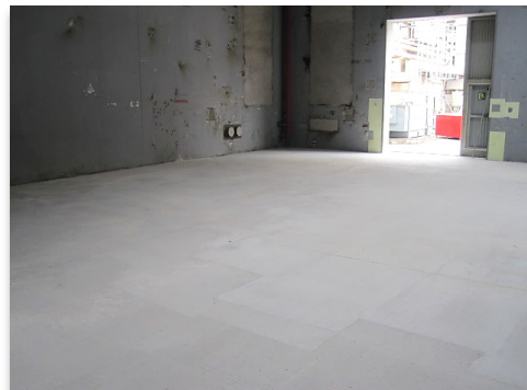
Diesel generator building converted into an auxiliary storage area.
