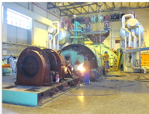
Dismantling of the turbine components.
