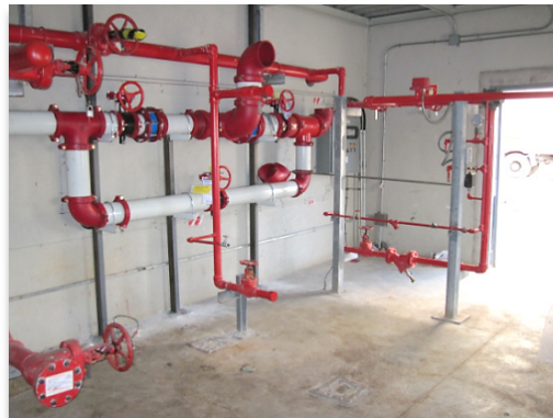
Fire protection system modification.
