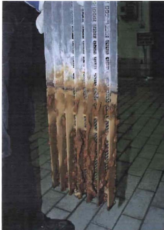
Figure 5-15: Hot-dip Galvanized Step Grating after having been Submerged in Borated Water for 2 Years.
