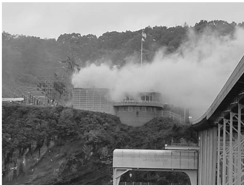
Fig. 3.10-2 Smoke from a cable fire at a non-nuclear power plant
