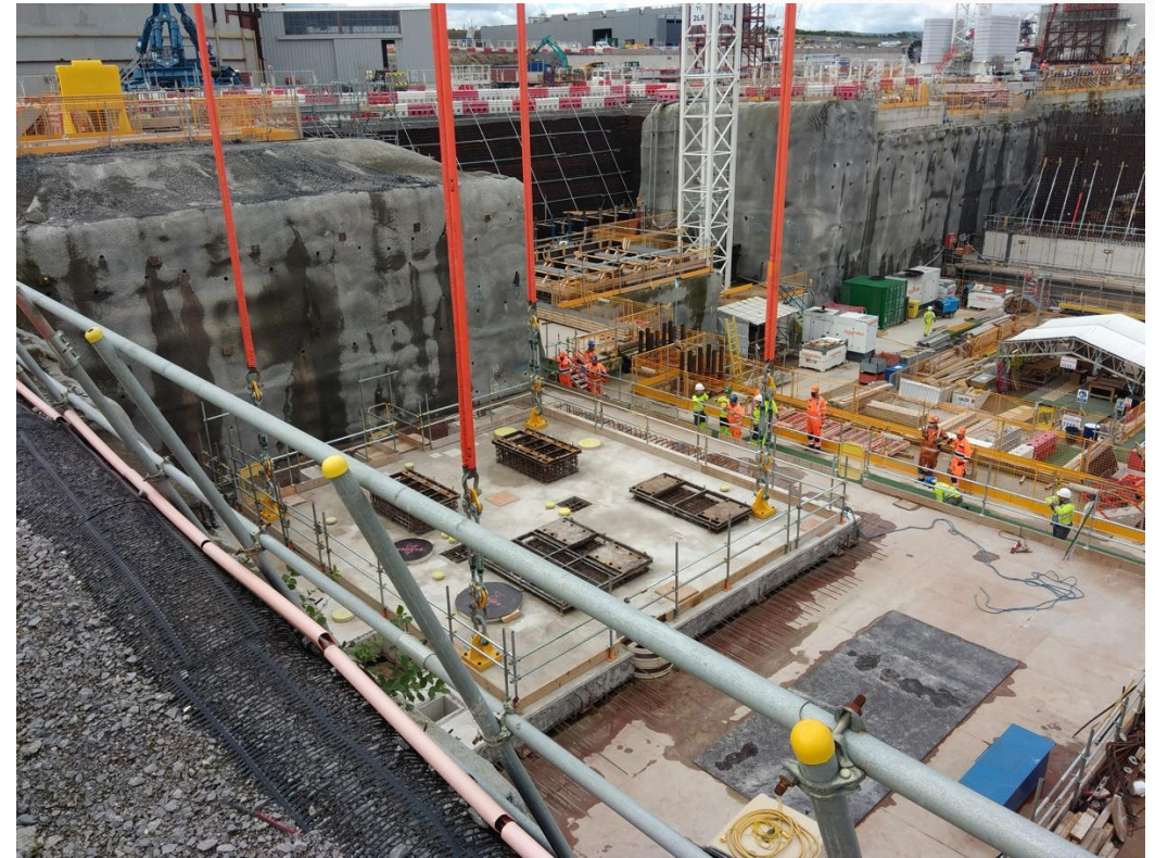
Photo: Lift HL1-02 Precast Slab – 18 Aug. 2020
