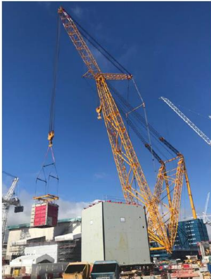
Photo: Lift ASG tank HL1 Unit 1 – 17 May.2021
