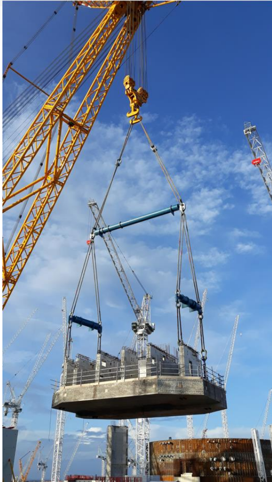
Photo: Lift South Precast Slab -2.30 HR-Unit 1- 18 Dec. 2020
