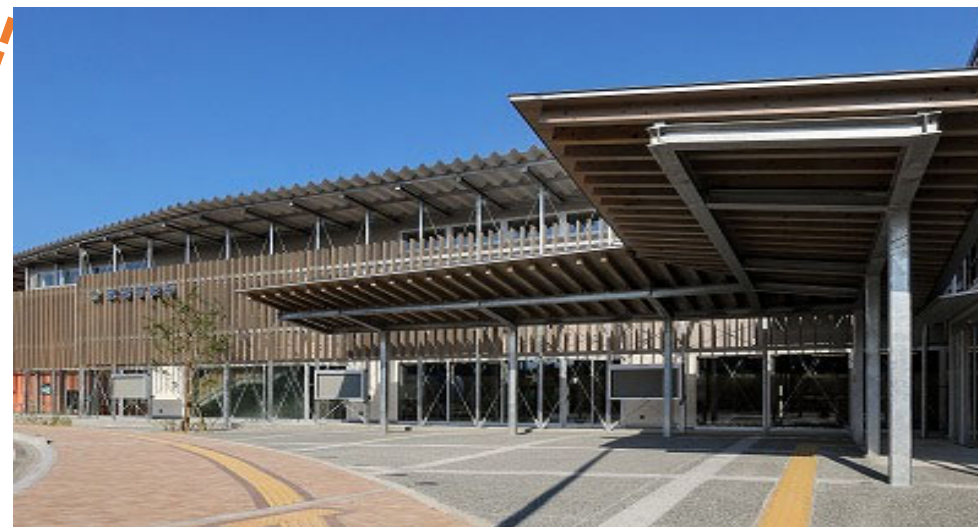
The Base area in Futaba Town where the Fukushima Daiichi NPS is located
