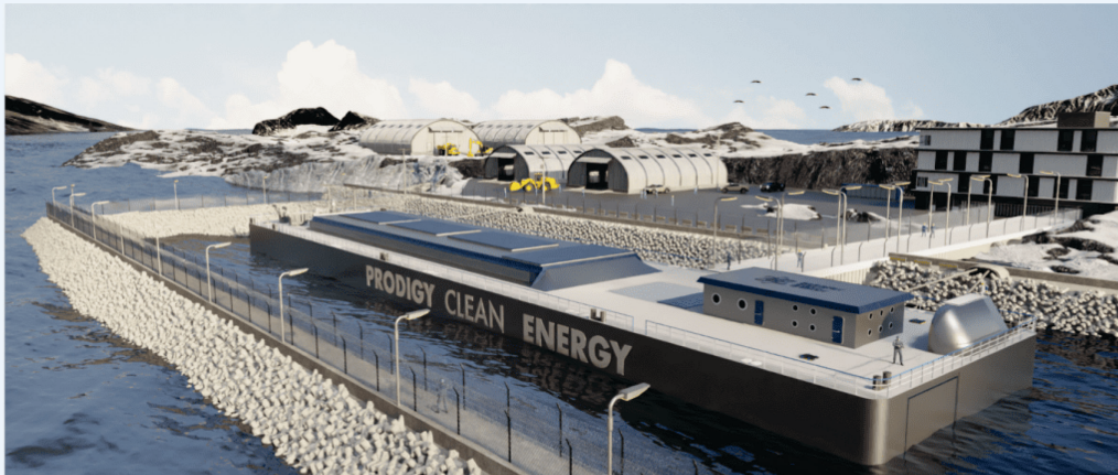
Figure 2.10: Rendering of the Prodigy Microreactor Power Station Transportable Nuclear Power Plant concept
